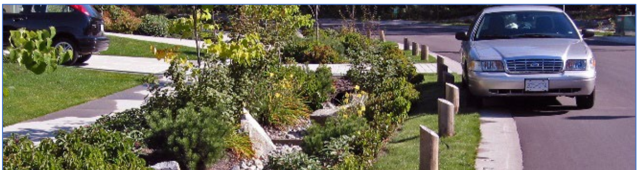
Figure 21: Storm water source controls – infiltration swale.
